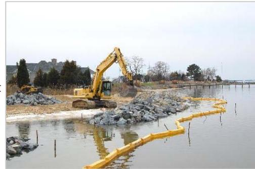
PHOTO BY CAROLYN SWIFT Local wetland restoration organization Environmental Concern should soon finish construction on the Cooperative Oxford Lab's "living shoreline." The project will protect the shoreline from water and storm erosion and create a habitat for Chesapeake Bay organisms.
